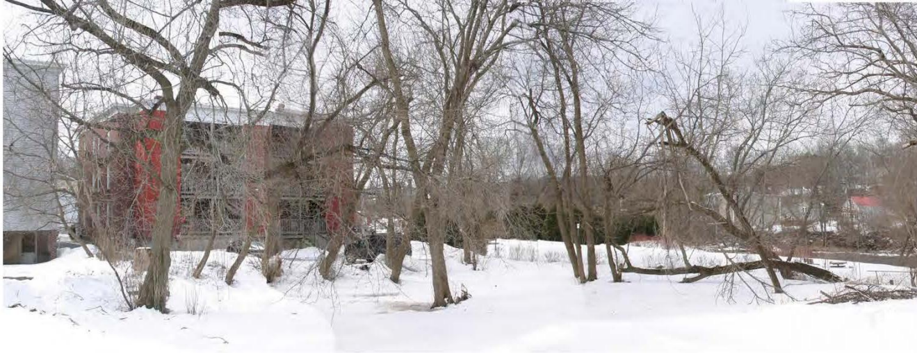
Figure 54: Riverway – Existing Conditions
